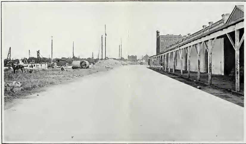
Hassam Pavement in the Warehouse District, Stockton, California
